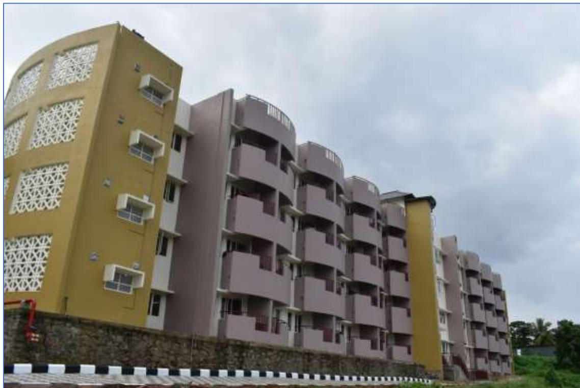
Hostel Number 3 (back view)
