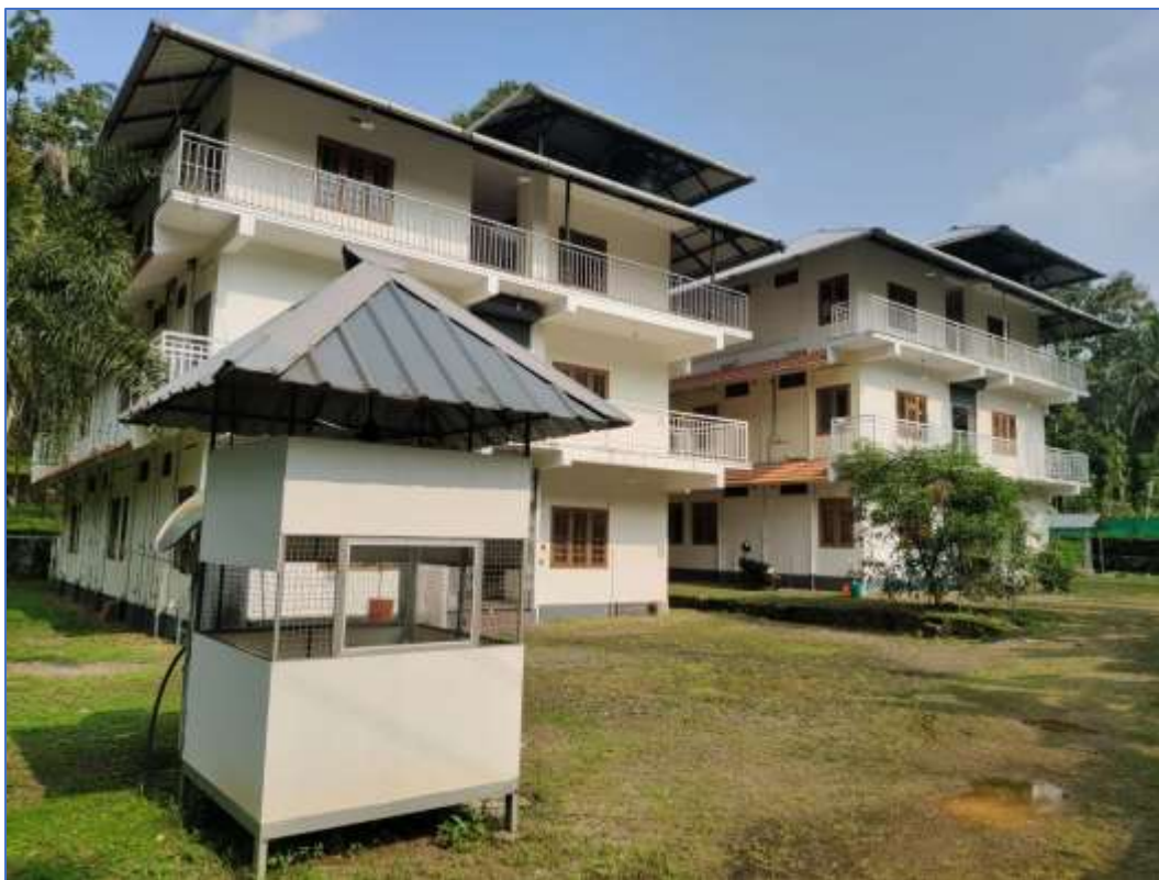
External Hostel – Block 1 & II – With Attached Bathrooms
