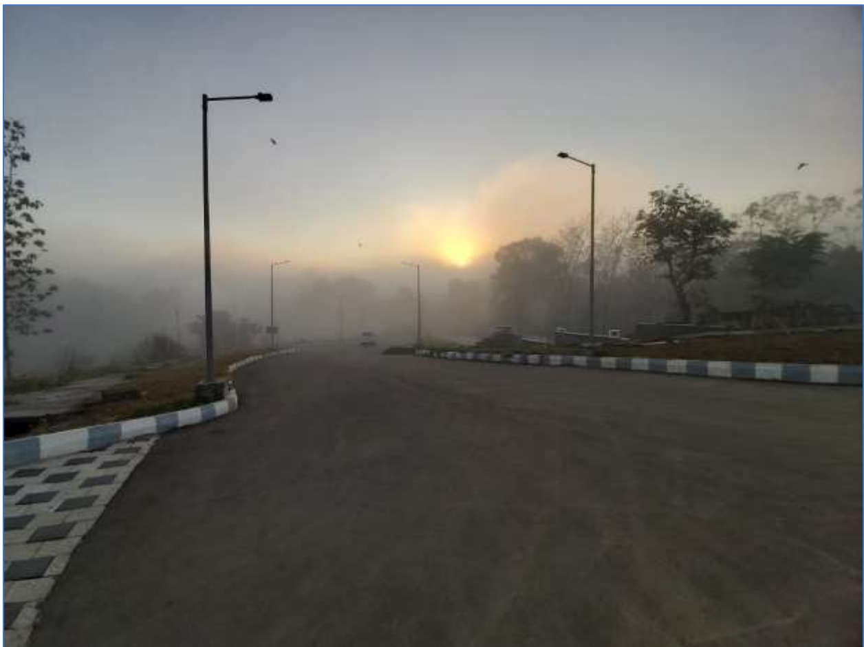
Roads inside the campus - Early Morning View
