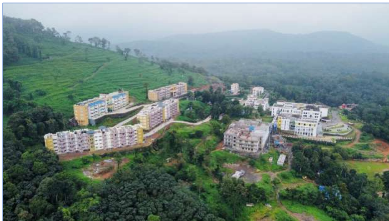
Arial View of entire IIIT Kottayam campus using Drone Camera (13 Nov 2022)
