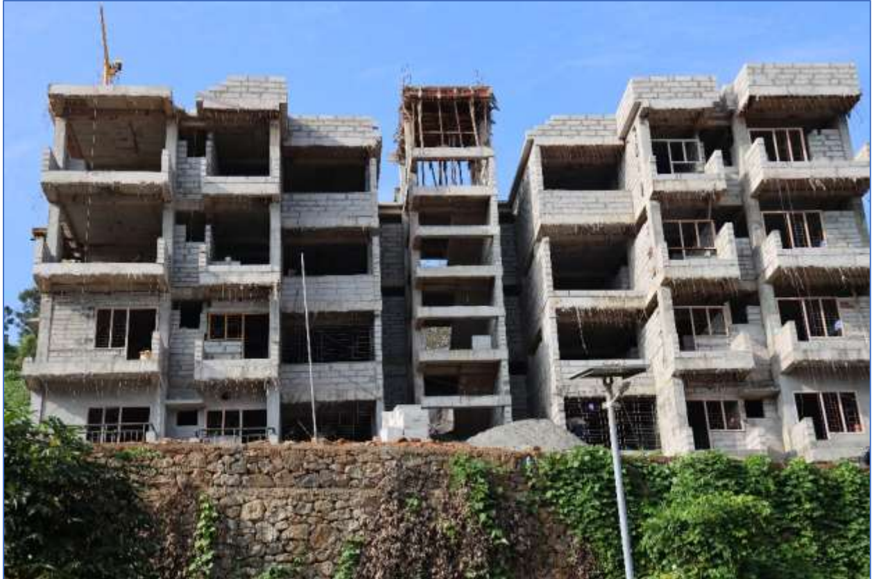
28 Staff Quarters 2 nd Building – Under Construction – Through Internal Revenue Generation (IRG) (on 05 Feb 2024)
