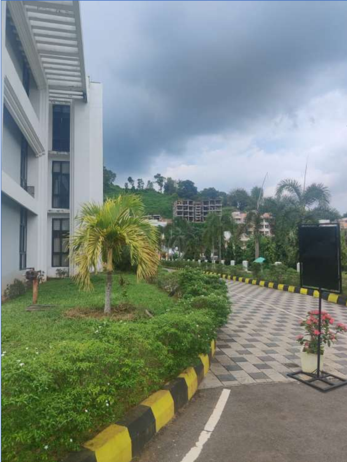
28 Staff Quarters Long Distance View Both the Buildings– Under Construction – Through Internal Revenue Generation (IRG) (on 02 Oct 2023)
