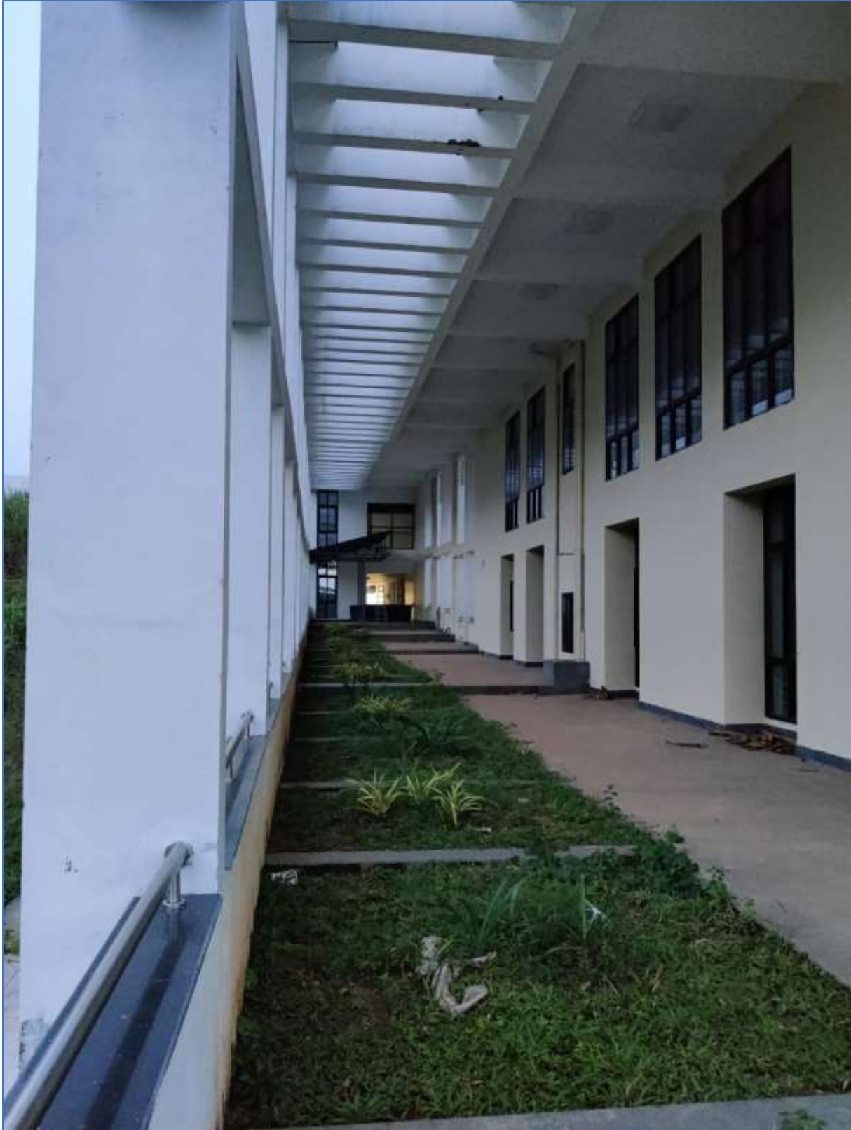
Passage between Academic Block 1 and Administrative Block
