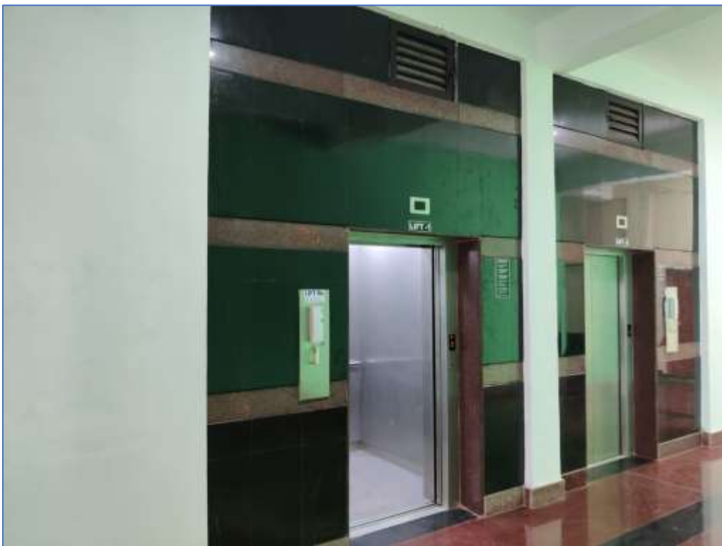
Lift – Administrative Block
