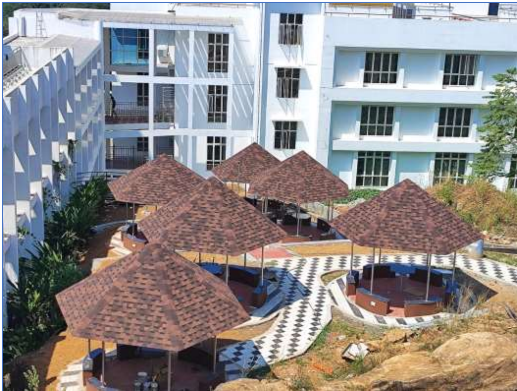
New Cafeteria - Under Construction - Through Internal Revenue Generation (IRG) (29 Feb 2024)
