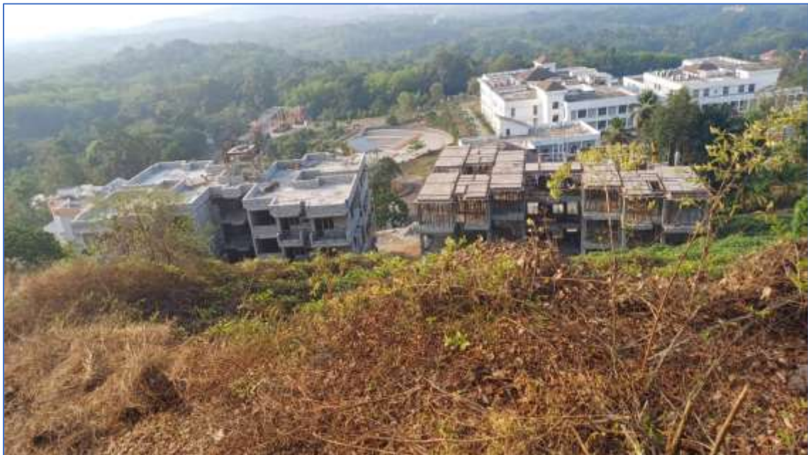
28 Staff Quarters Top View Both the Buildings– Under Construction – Through Internal Revenue Generation (IRG) (on 27 Feb 2024)
