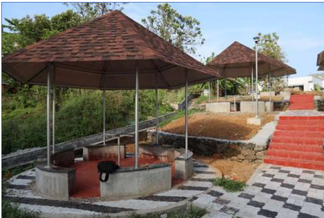
New Cafeteria - Under Construction - Through Internal Revenue Generation (IRG) (05 Feb 2024)
